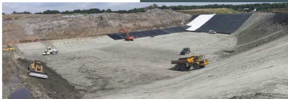
Landfill cell being engineered
